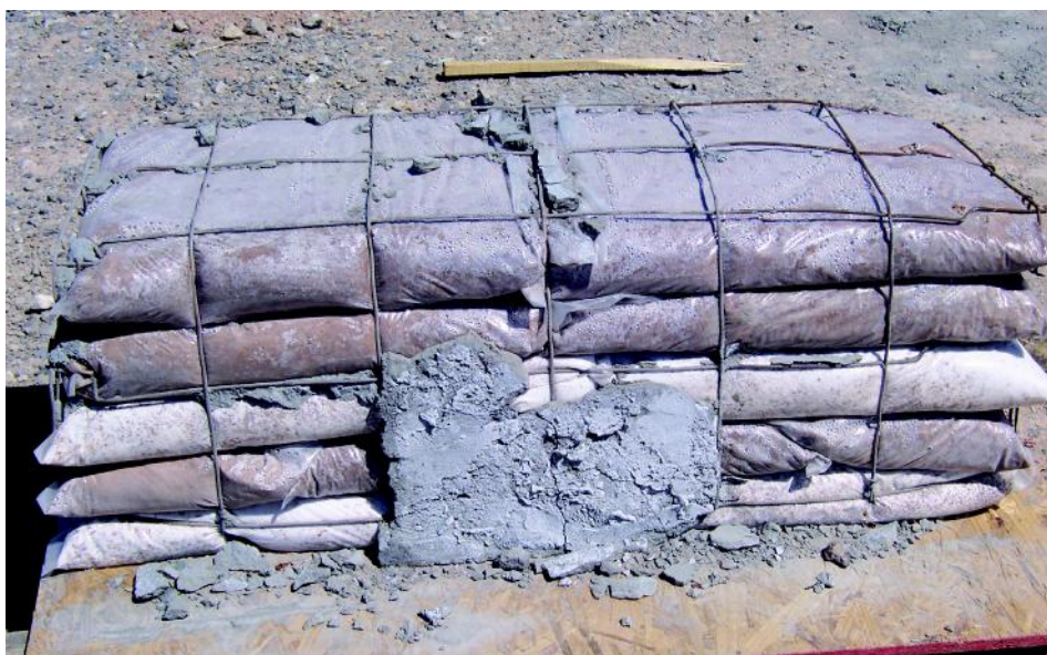
The home's construction materials included sandbags (adobe style), steel mesh and cement.
